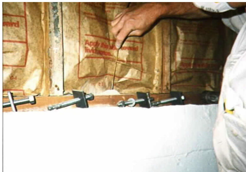
Figure 6 Mechanical anchor bolts for connecting the sill plate to the foundation wall. Note that square washers are required. (Photo from Ben Emam, Amazon.com)
