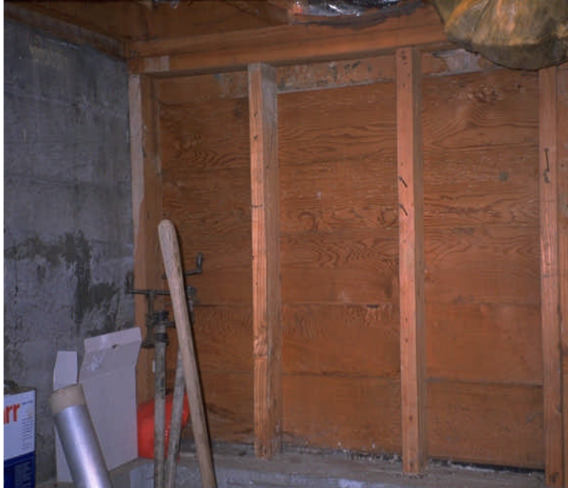
Figure 8 Pony wall without structural panels to strengthen the wall to prevent excessive side sway that may lead to collapse of the wall. Note the sill plate is embedded into the foundation wall. (Photo by Linda Noson, AGRA Earth & Environmental)
